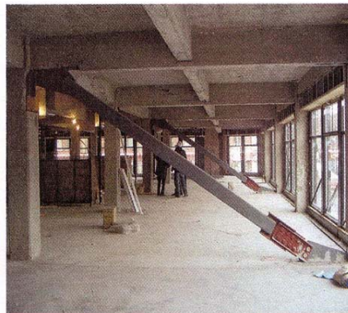
Figure 2 One-way diagonal brace with Pall friction damper
