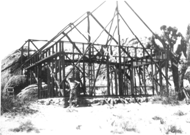
Figure 2: Historic photo of construction of the Antelope Valley Indian Museum
